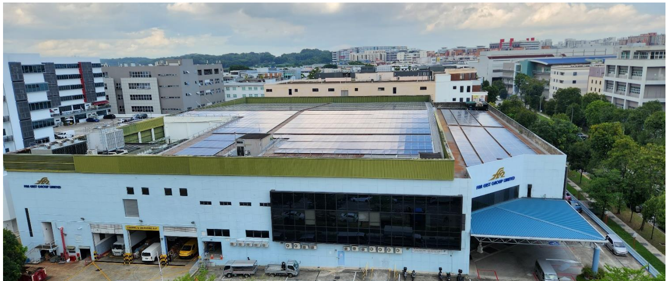
Regional headquarters covered with solar panels
