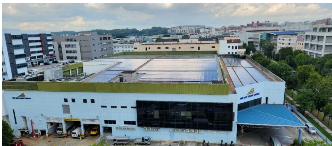
Regional headquarters covered with solar panels
